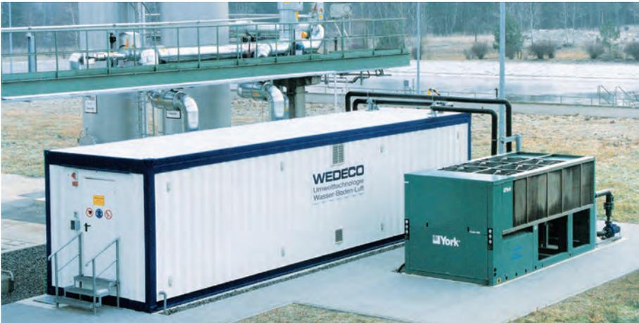
**Ozone Generator with an Oxygen Plant and Chiller System**
