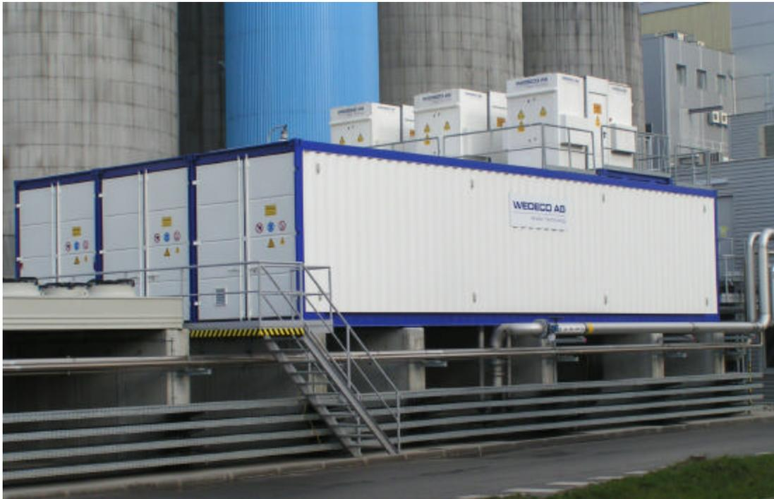
A CONTAINERISED OZONE SYSTEM IN A PULP MILL
