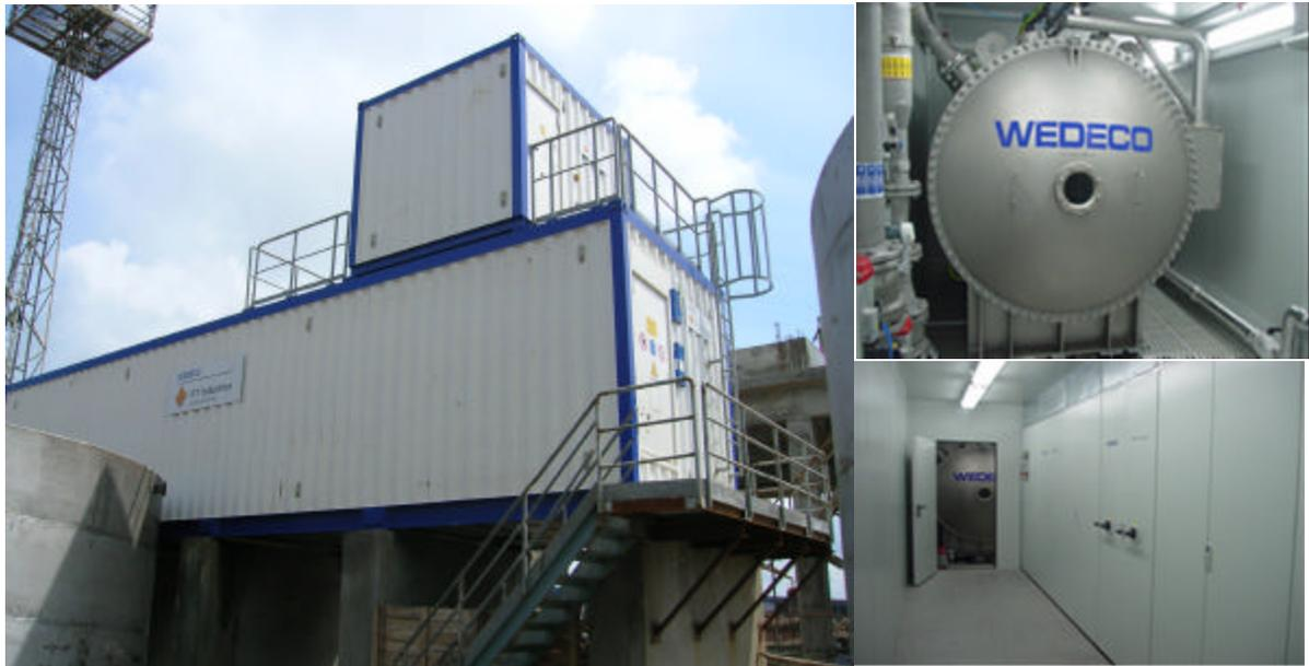
Figure: Worldwide largest single containerized Ozone Generator / ITC pulp mill.
